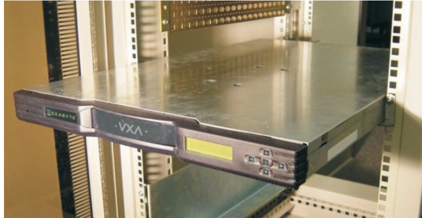
Figure 10. Placing the autoloader on the rails
